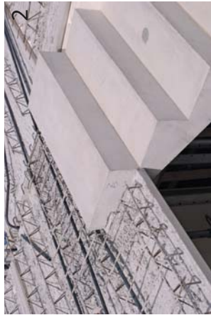
Emfil Stair connected to Emfil Slab
