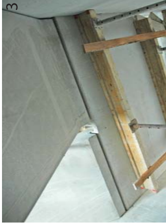
Emfil Stair connected to Emfil Slab
